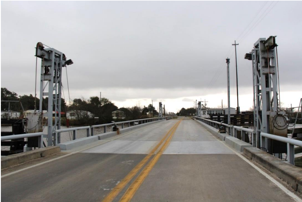
Condition Photo 1: Overview of pontoon swing span.
