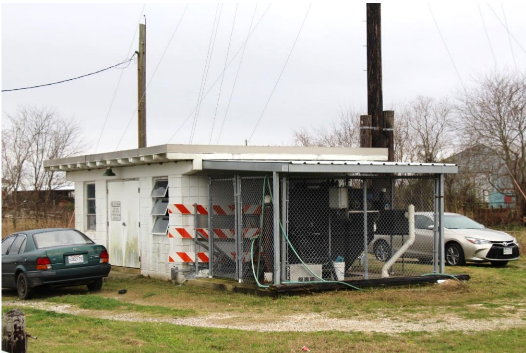
Historic Fabric Photo 4: Generator house.
