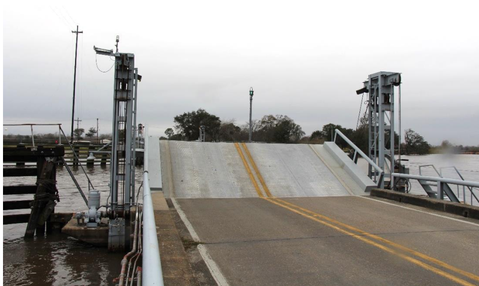
Character-defining Feature Photo 4: Design and construction of a pontoon swing span including the pivot arm, the two approach apron lift spans, and the four lift towers. The approach apron lift plate shown raised vertically.
