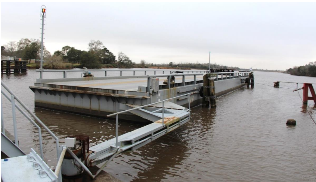
Character-defining Feature Photo 2: Design and construction of a pontoon swing span including the pivot arm, the two approach apron lift spans, and the four lift towers. The main swing span (open), showing the pontoon and pivot arm.
