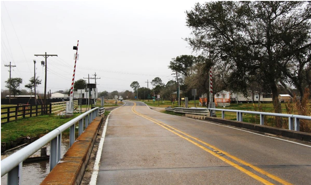
Historic Fabric Photo 1: Concrete approach spans.
